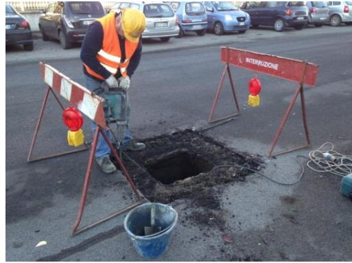
Removal of material around the frame
