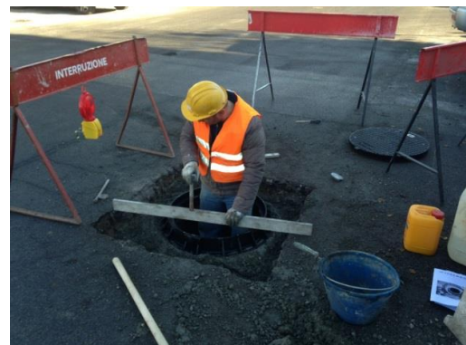
Frame adjustment to road level
